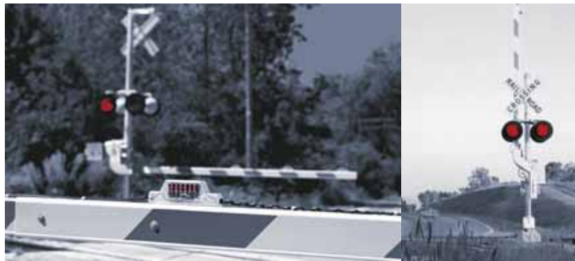
Picture 6: Signaling at a crossing gate
