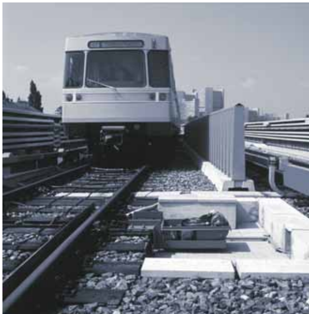
Picture 4: Points Machine along the tracks.
