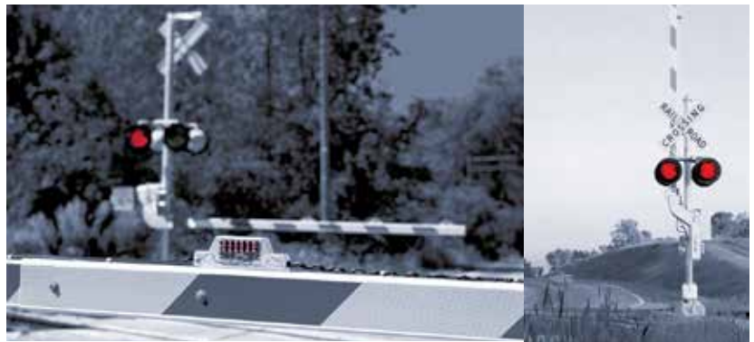
Picture 6: Signaling at a crossing gate
