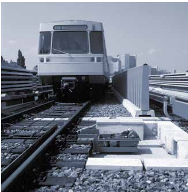
Picture 4: Points Machine along the tracks.
